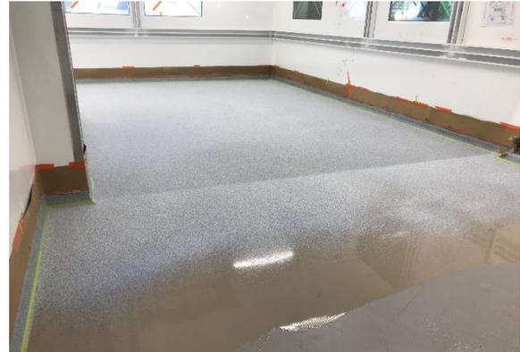
Following this the first MMA membrane is poured out on the level floor - this is a self-levelling liquid product, approximately 1.5mm thick. Next, a wearing layer is poured, this is slightly thicker at 2mm and now things have to move quickly as the multi-coloured fleck finish must be applied before it dries. Workers hand cast the fleck, so applying a consistent spread requires a practised technique. After curing, any excess fleck is collected up to be used again.
